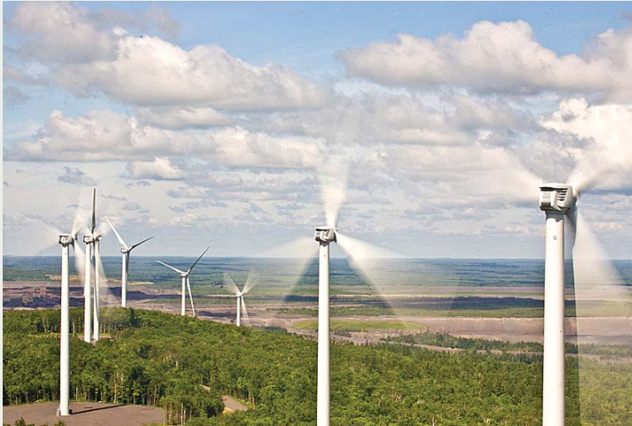
Minnesota Power wind turbines producing renewable energy
