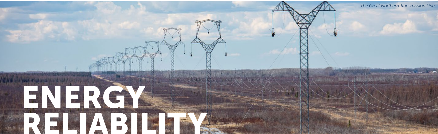
The Great Northern Transmission Line
