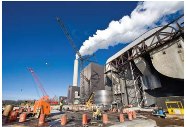
Emission control work proceeds at Boswell Unit 3
