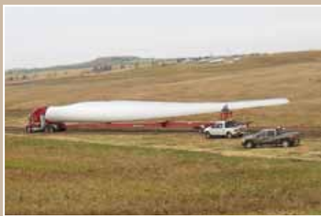
Wind blades arrive at Bison construction site.
