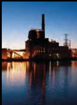
Duluth Steam District #2 is located at the Hibbard Energy Center in Duluth, Minn.
